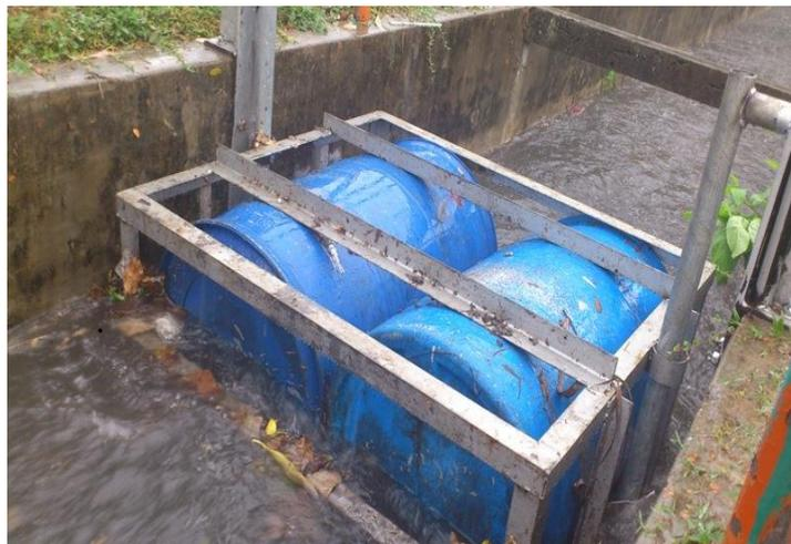
Figure 4: Floating Rubbish Trap when operation
